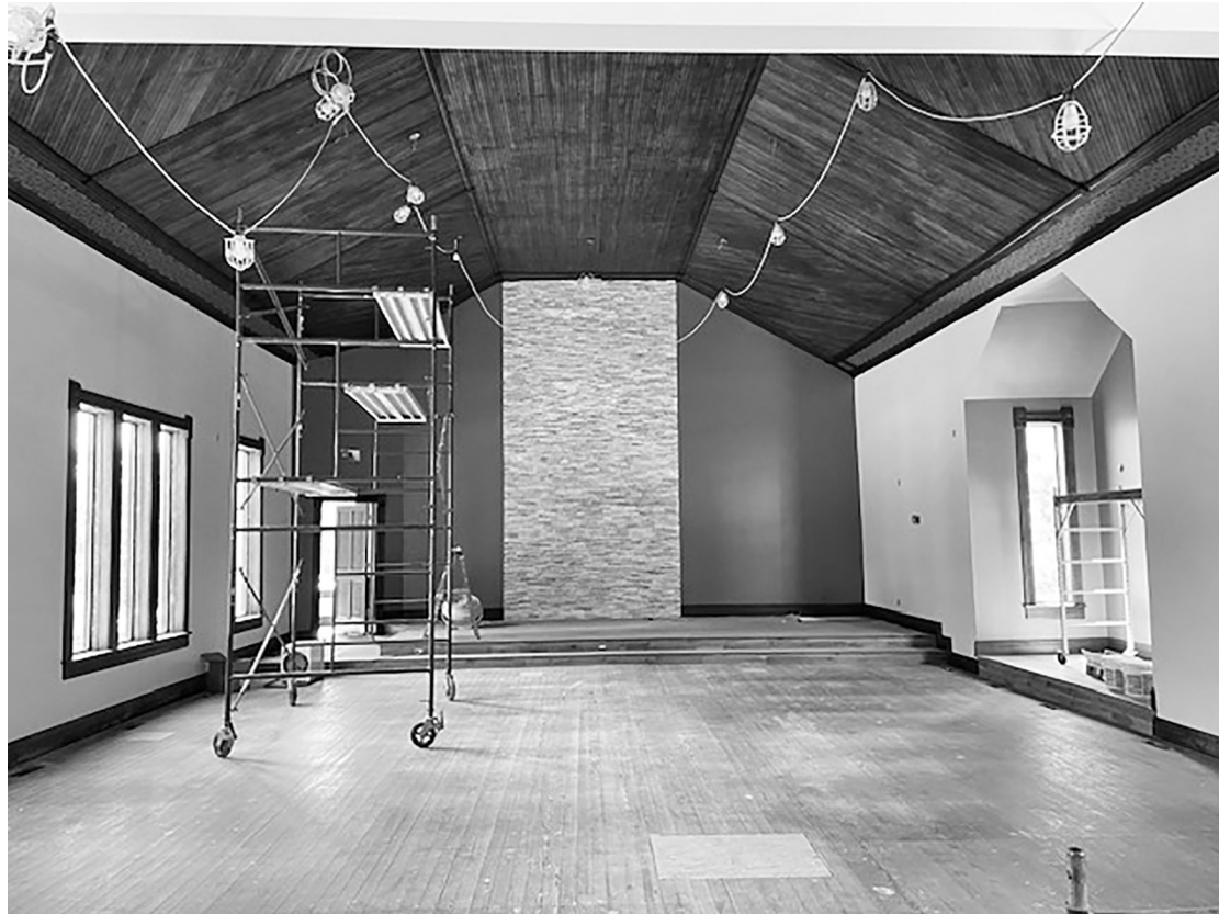
This Sept. 14 photo of the inside of St. Jude Thaddeus Church in Mokane highlights the vaulted ceiling, which had been hiding behind a drop-ceiling for decades. Repairs and renovations are nearing completion to keep the 128-year-old church sound and viable for new generations. — Photo by Heather Murphy
